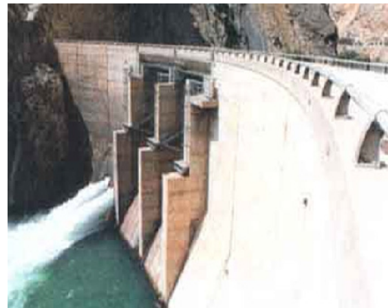
Fig. 1. Location of Amir Kabir Dam.
