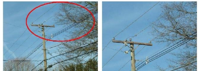
**Fig. 1.** Potential HIF Due to Tree-Limb Contact.
