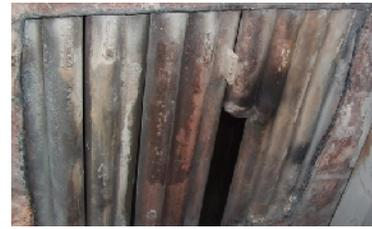
**Fig. 3.** Bank Tubes of Boiler-I SGP NFL Naya Nangal.
