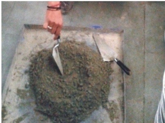
Fig. 5. Preparing mix of M-20 concrete.
